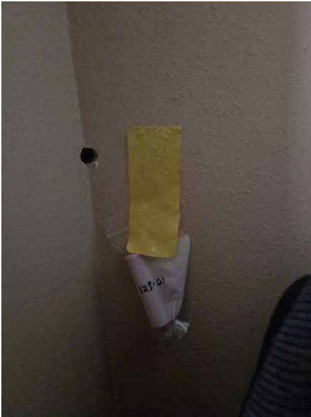
Sample 123-01 Typical Drywall & Joint Compound Sample
