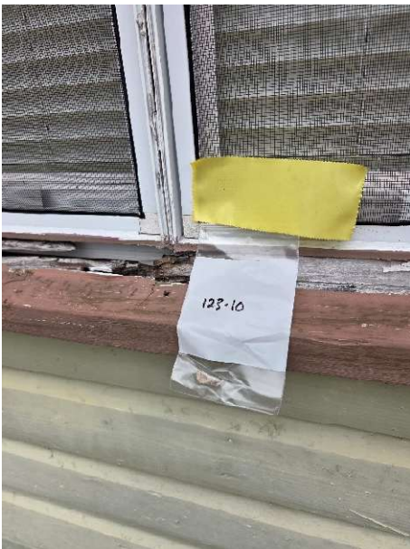
Sample 123-10 Typical Exterior Caulking Sample
