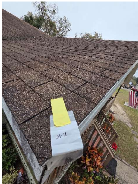
Sample 123-13 Asphalt Shingle Roofing Sample
